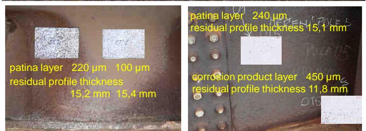
Figure 5 – The examples of damage of weathering steel structures
