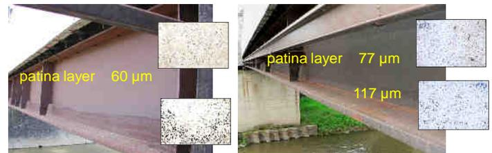
Figure 3 – The specific affected areas above low flange – the same bridge evaluated in 2002 (left) and 2009 (built 1986)
