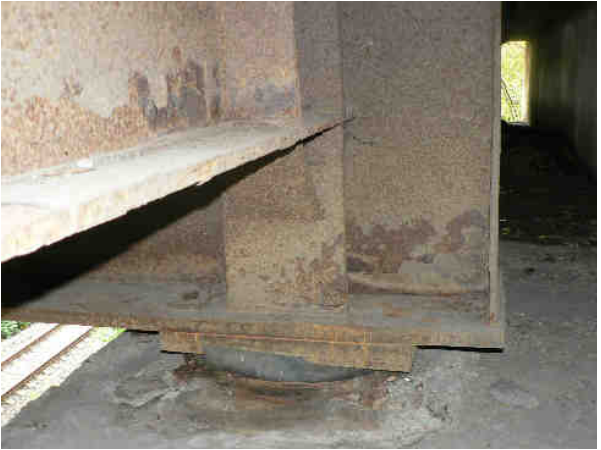
Figure 4: Examples of rust layer above bottom flange
