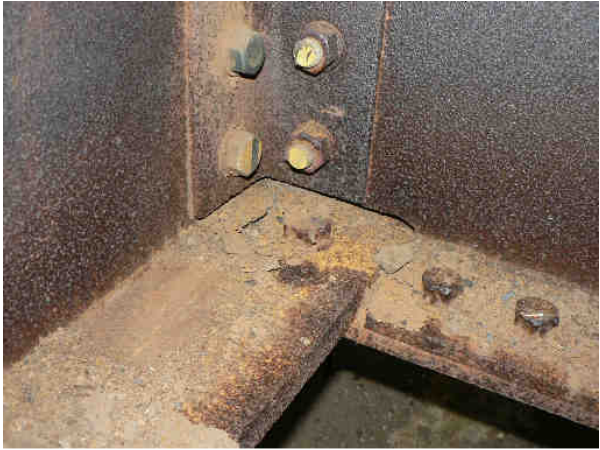
Figure 4: Examples of rust layer above bottom flange
