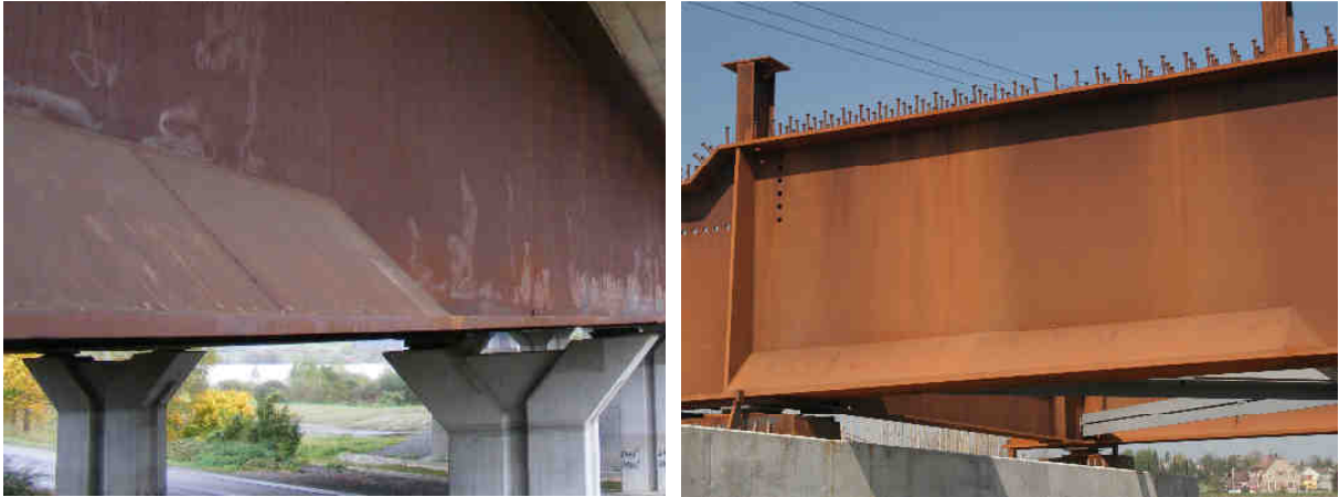
Figure 5: New design of low flange element
