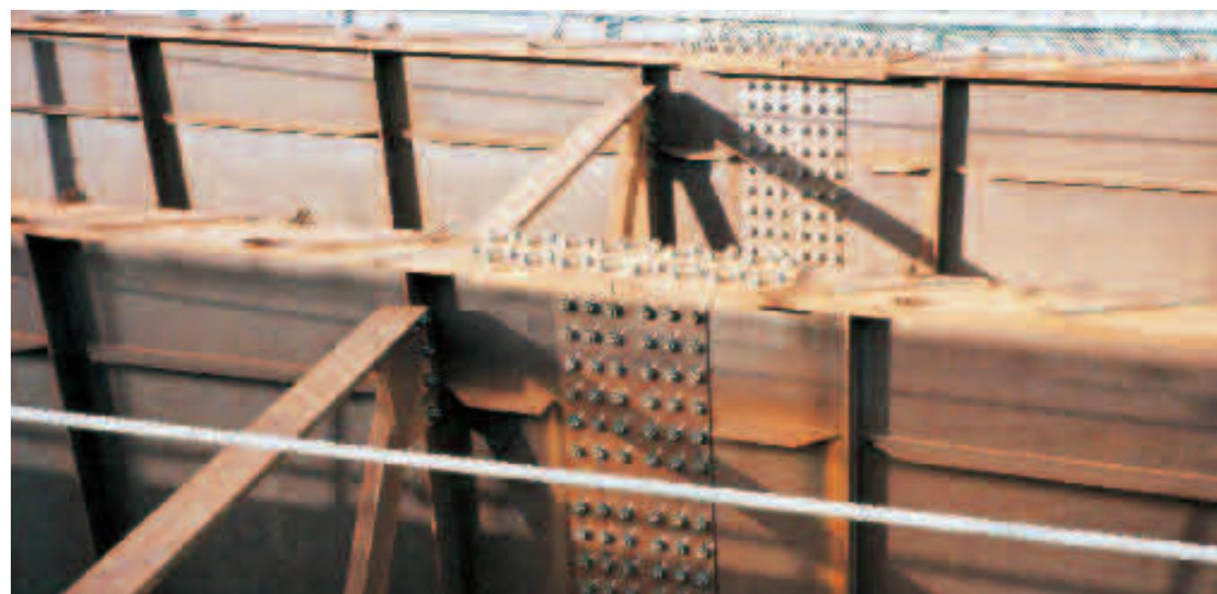
Coastal weathering steel (3%Ni-type) is applied at the left side of the spliced portion and the conventional weathering steel at the right side.
