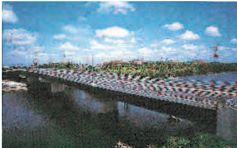
Coastal weathering steel (5% Ni-type) was used for parts of Shin-Nittetsu Minami Ohashi Bridge.
